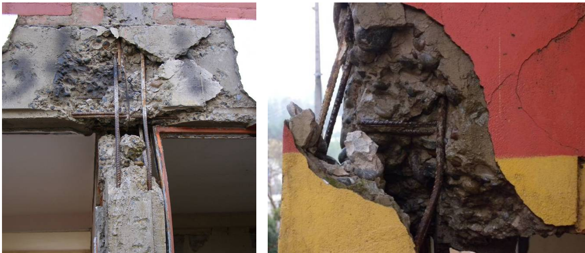
Figure 23. Buckling of longitudinal reinforcement due to inadequate confinement in the end zones of RC tie-columns (Brzev et al., 2010).
