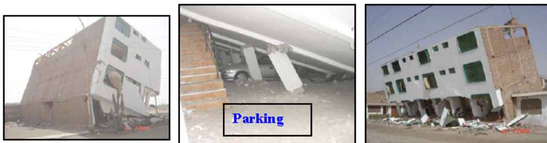
Figure 21. Collapse of a four-story confined masonry building in the 2007 Pisco, Peru earthquake (San Bartolomé and Quiun, 2008).
